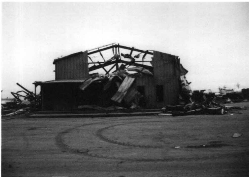
Figure 6.8 A Metal Building System as described by the Damage Classification guide. Damage to this building resembles the damage to the metal garage in Figure 6.7
