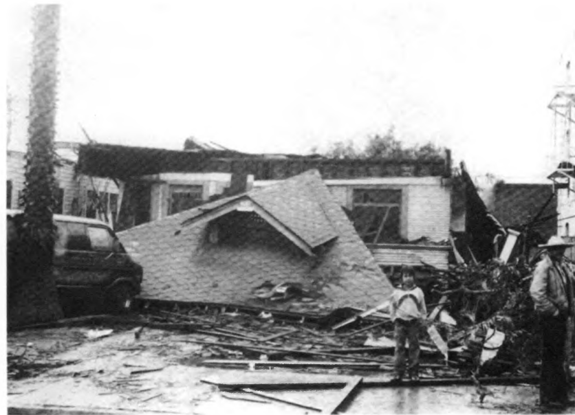
Figure 6.18 Collapse of entire roofing structure, house located near the Convention Center
