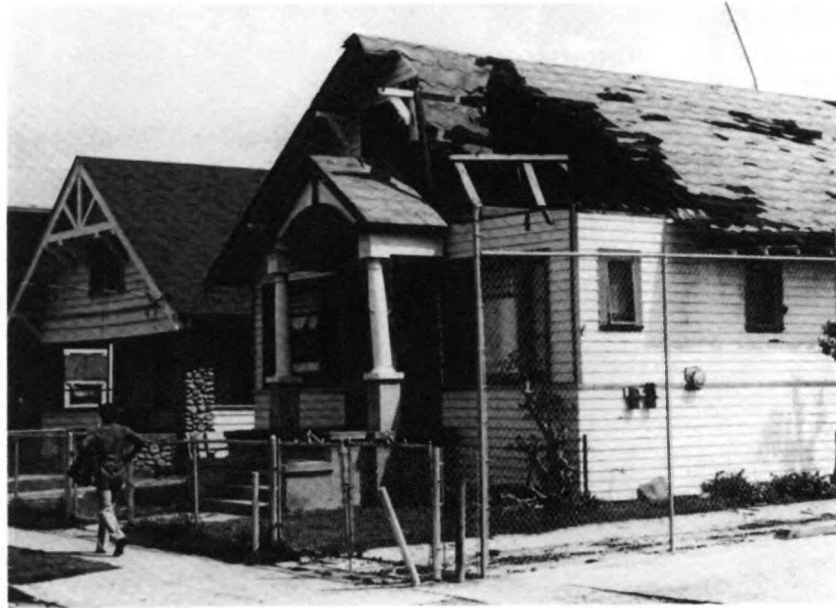
Figure 6.17 Section of roof removed from house located near the Convention Center
