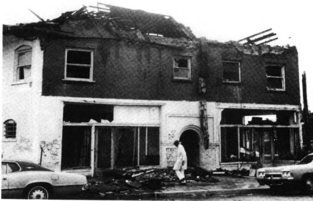
Figure 6.16 Damage to storefront windows. Collapse of masonry parapet and part of roof.
