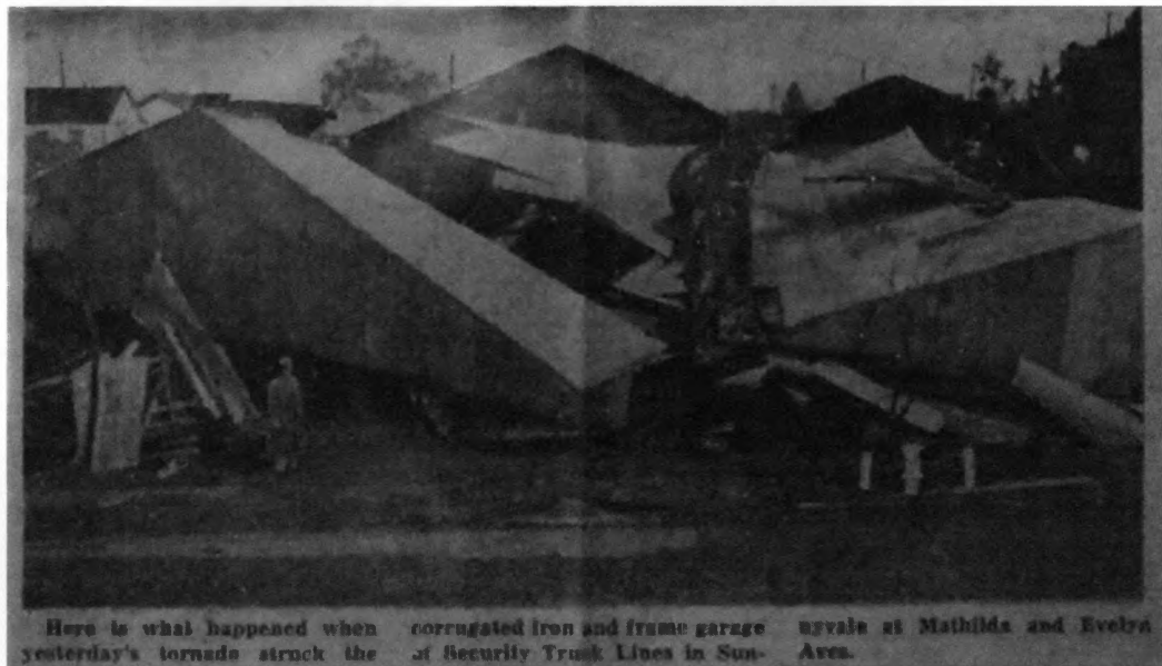
Figure 6.7 Corrugated iron and frame garage in Sunnyvale, CA knocked down on January 11, 1951.
