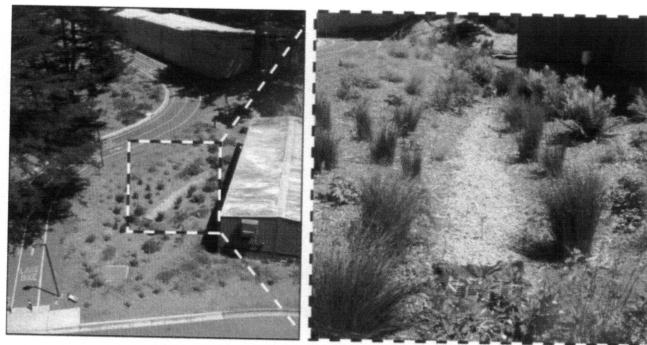
Figure 2. Photographs of the infiltration trench at the San Francisco State University (SFSU) low impact development (LID) research network. Modified from Newcomer et al., 2014.
