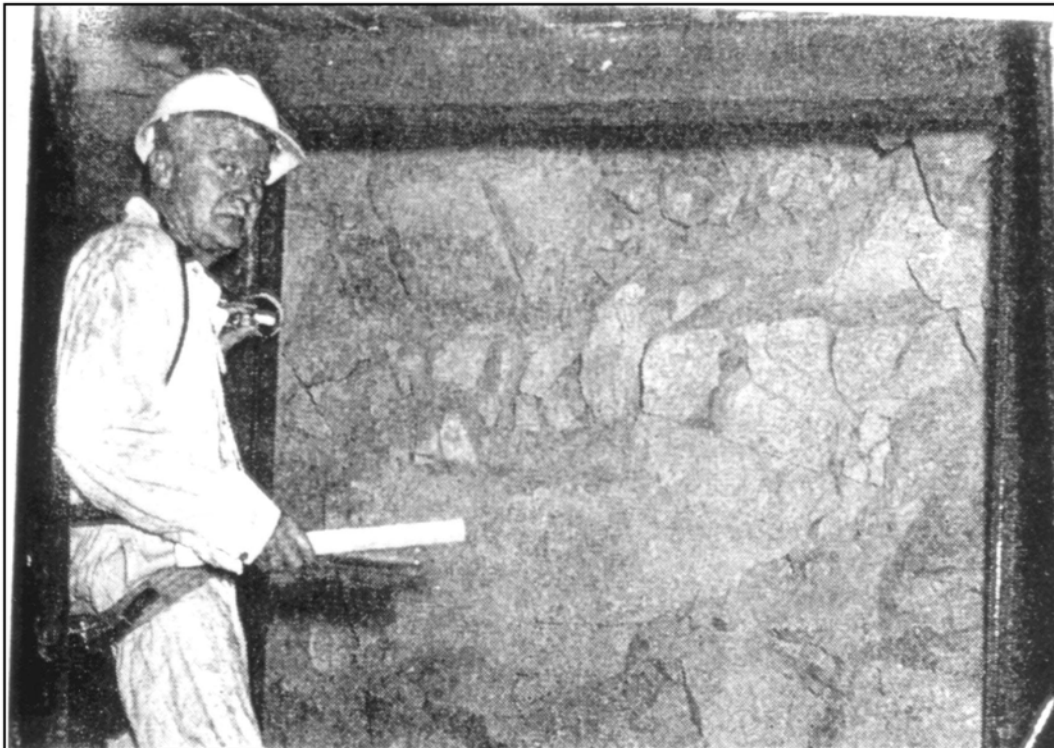
Fractured rock from PILE DRIVER chimney as viewed from side tunnel 600 feet below the surface. LLNL photo.
