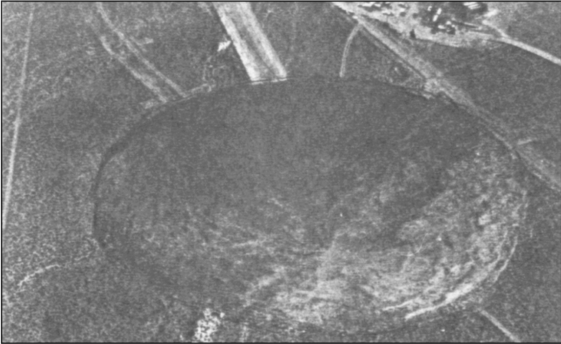
HUTCH subsidence crater. LLNL photo.
