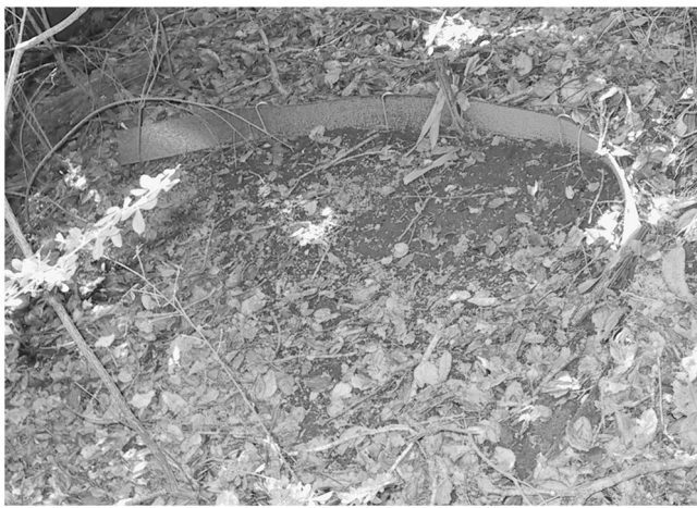
Figure 10. Downslope movement of leaf litter and soil. Note the exposed ground below the barrier.
