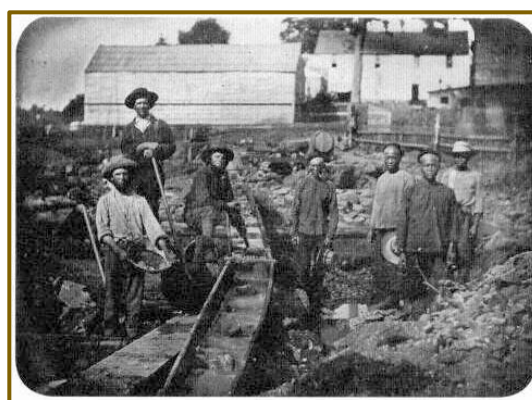
Figure 7: Photo shows sluices that gold miners used to obtain gold flakes from sediment recovered by hydraulic mining by adding mercury to the bottom of the sluice. Photo source: Rawls and Orsi, 1999
