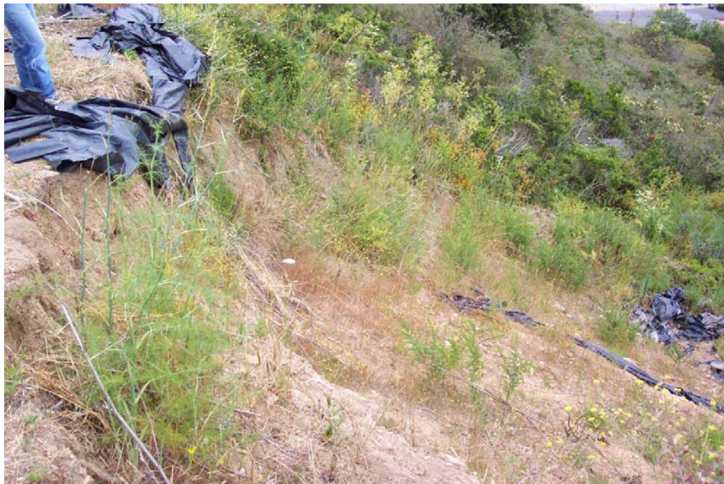
Figure 99: Erosion control tarps washed downslope of trail on landslide deposit. (Point 4 on Figure 95).
