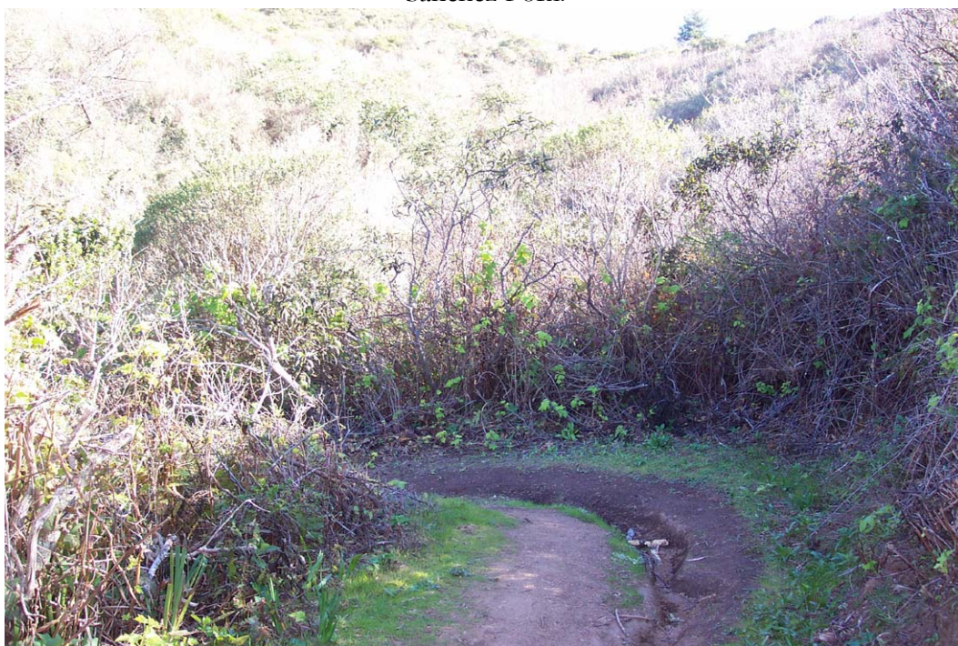
Figure 30: Concentrated flow creating surface erosion and increasing the effective drainage density along the Hazelnut Trail draining to South Fork.
