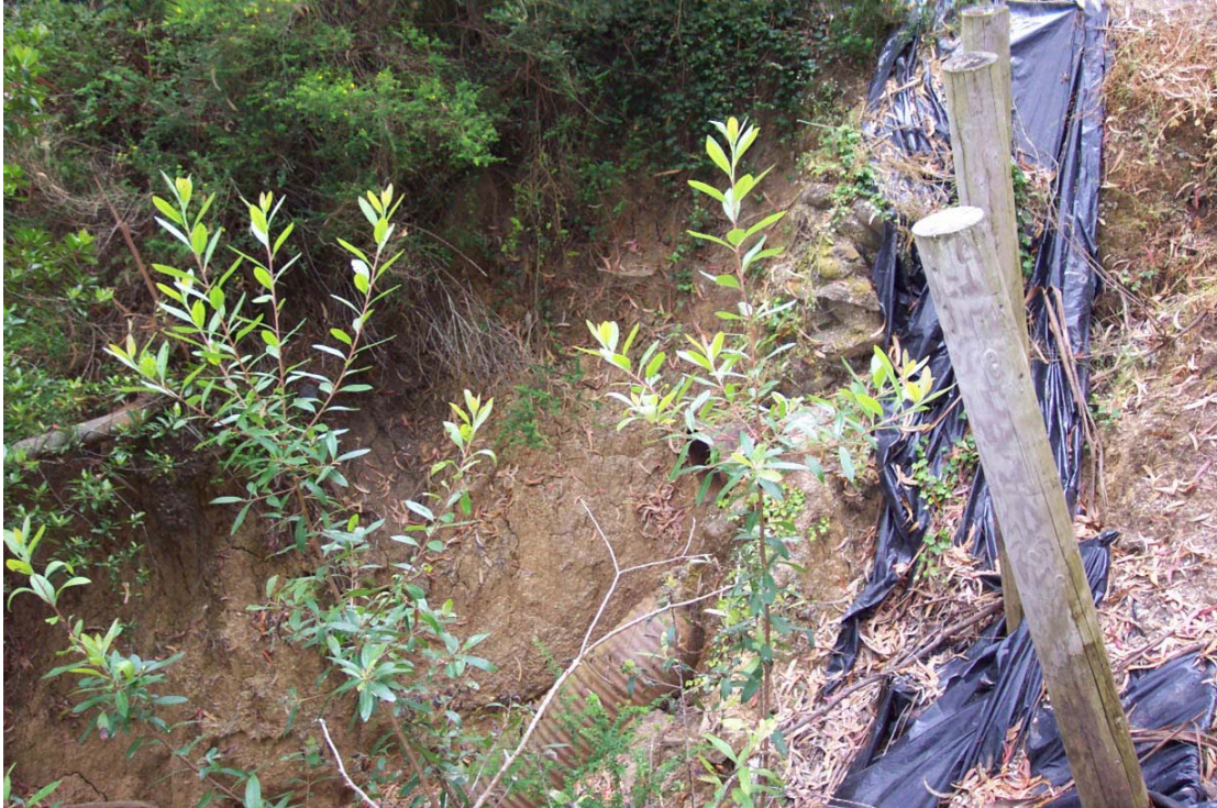
Figure 96b: Severe gully in drainage downslope of paved Coastside Boulevard. Same gully as shown in 96a taken 8 months later after one complete rainy season. Tarps have washed downslope and culvert has broken and moved partially downslope (Point 1 on Figure 95).
