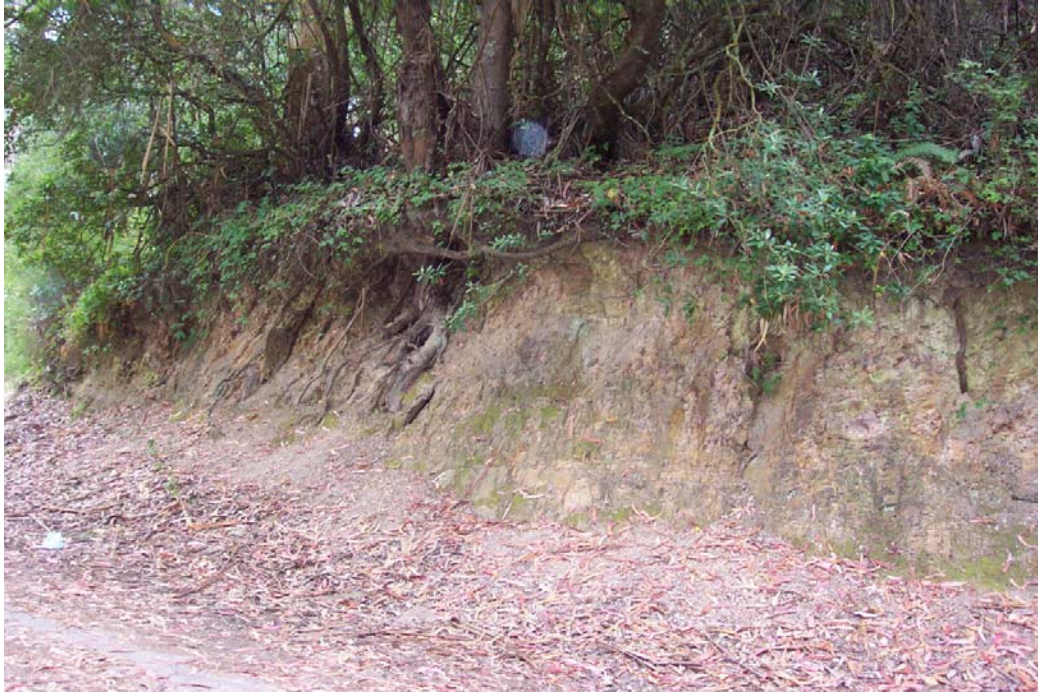
Figure 98: Undercut vegetation and exposed tree roots on upper trail cut along Coastside Boulevard (Point 2 on Figure 95).
