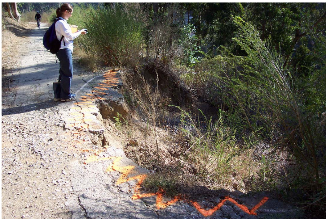
Figure 72a: Severe mass wasting and subsequent surface erosion downslope of Coastside Boulevard draining to Sanchez Fork (Point 1 on Figure 69).
