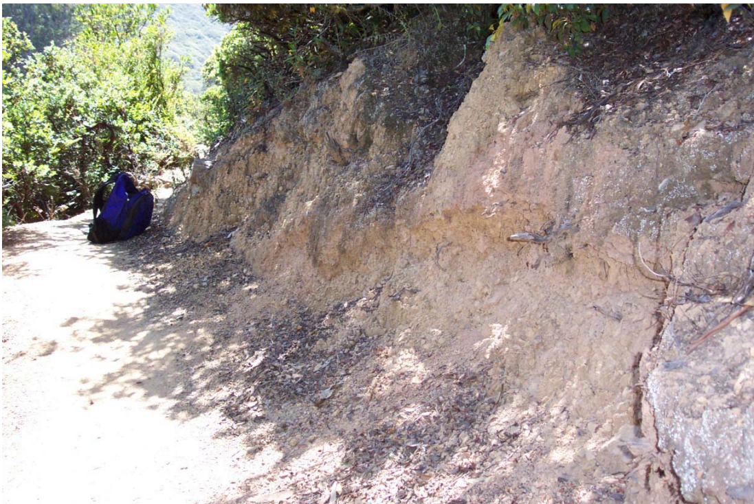
Figure 67: Surface erosion along Brooks Creek Trail (Line 4 on Figure 61).
