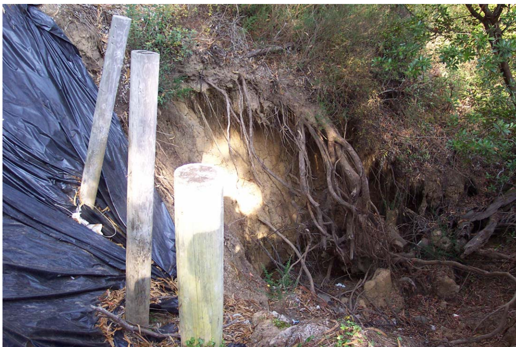
Figure 29: Severe surface erosion from concentrated Horton overland flow downslope of Coastside Boulevard, draining to a culvert draining to the storm drain network near Sanchez Fork.
