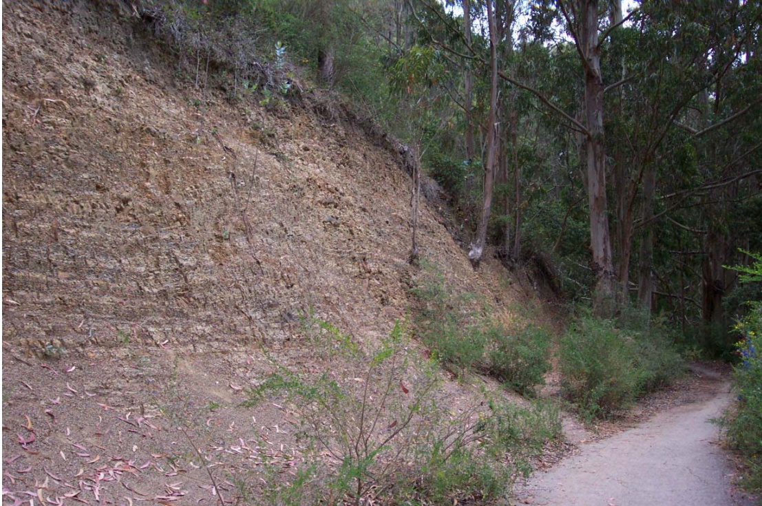
Figure 78: Trail cut eroded to bedrock with sediment accumulation along the base from surface erosion along upslope soils (Point 8 on Figure 71).
