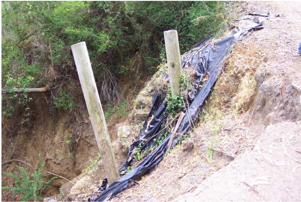
Figure 104: Ineffective erosion control structures. Tarps have washed downslope over the sandbags supporting the trail in just one rainy season.
