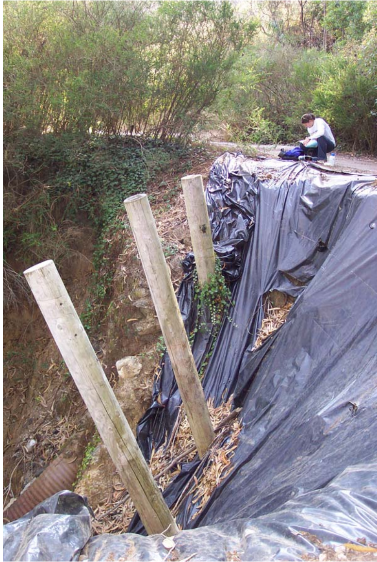
Figure 96a: Severe gully in drainage downslope of paved Coastside Boulevard (Point 1 on Figure 95).
