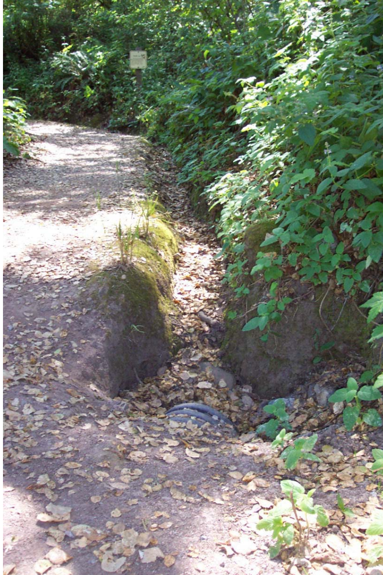
Figure 62: Fluvial erosion along a ditch from ephemeral drainage along uphill section of lower Hazelnut Trail (end of Line 1 on Figure 61).
