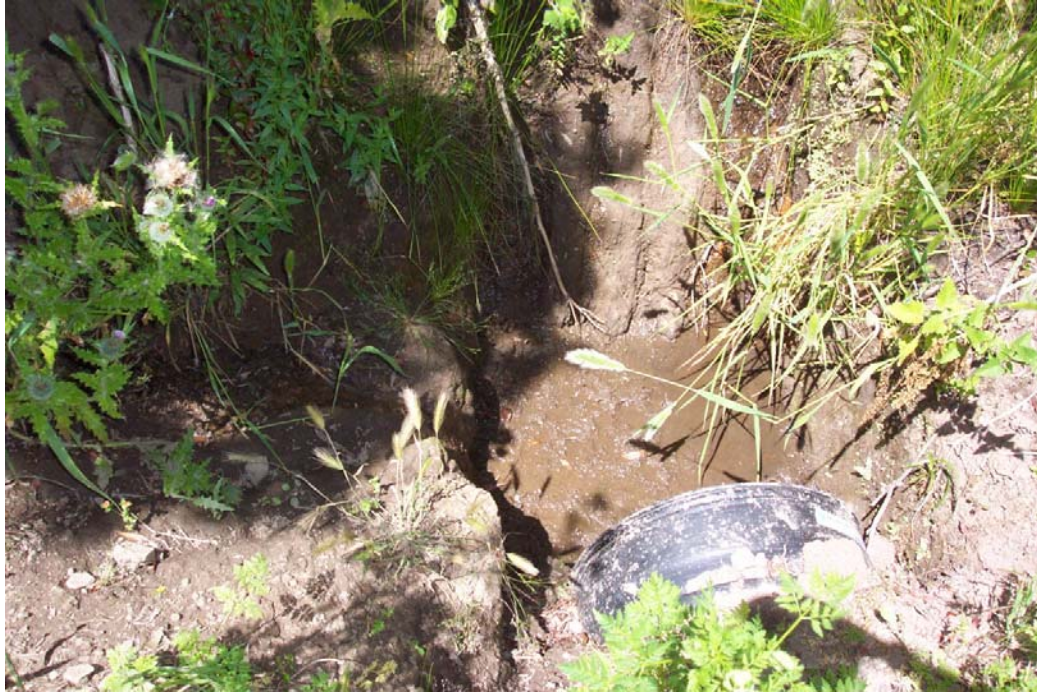
Figure 83: Sediment in excavated culvert draining directly to stream along the trail upslope from the Shamrock Ranch (end of Line 8 on Figure 79).
