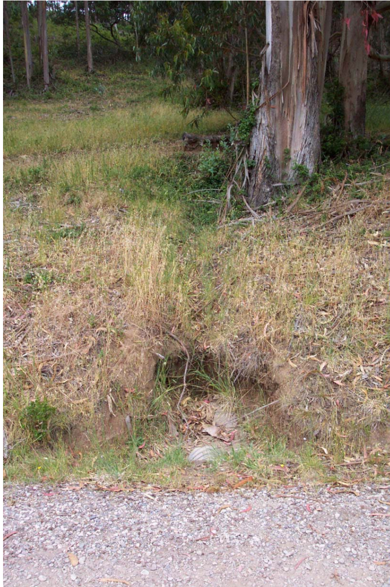
Figure 57: Incision at culvert from uphill ephemeral drainages (Point 6 on Figure 53).
