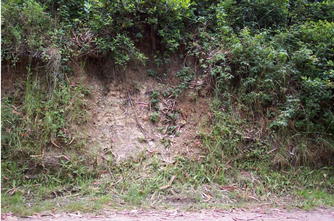
Figure 60: Surface erosion along an upslope roadcut draining to ditch and culverted under the road directly to the Middle/South fork (Point 1 on Figure 59).
