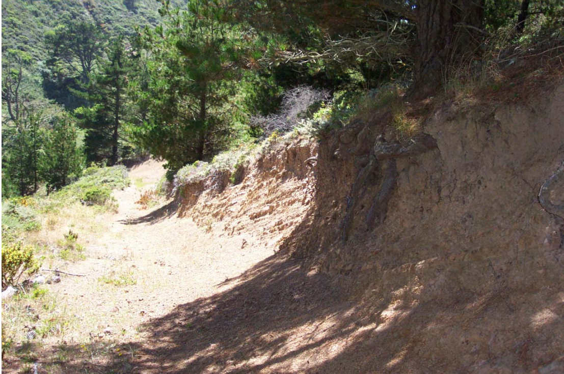
Figure 92: Erosion to bedrock exposing tree roots along upper trail cut. Upslope from eroded trail at line 1 on Figure 89 increasing the effective drainage where incision is initiated.
