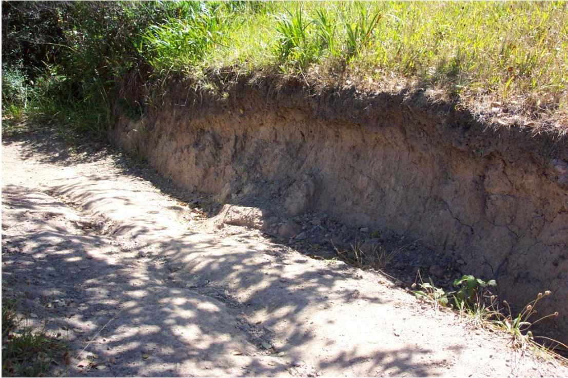
Figure 63: Surface erosion along uphill section of trail. Channel on inside where sediment deposits and in the middle of the trail (upper portion of Line 1 on Figure 61).
