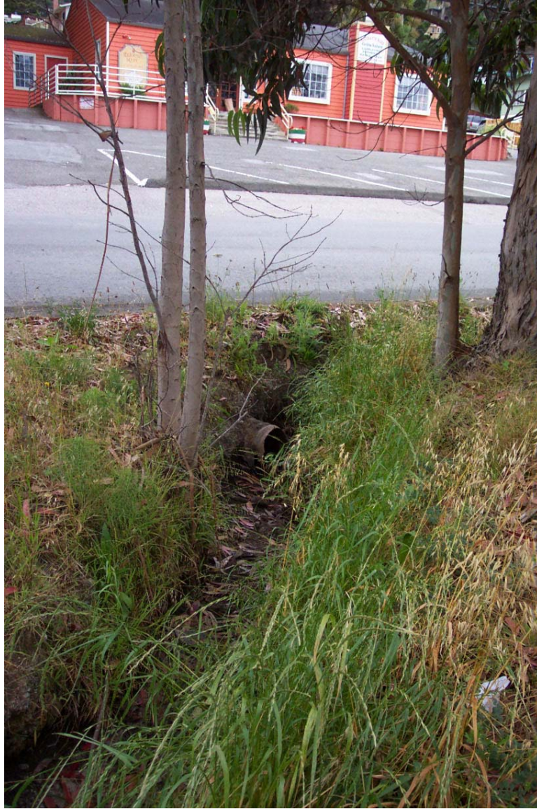
Figure 87: Channel incision from another culvert draining the urbanized hillslope and accumulated flow from culvert at Point 2 on Figure 85.
