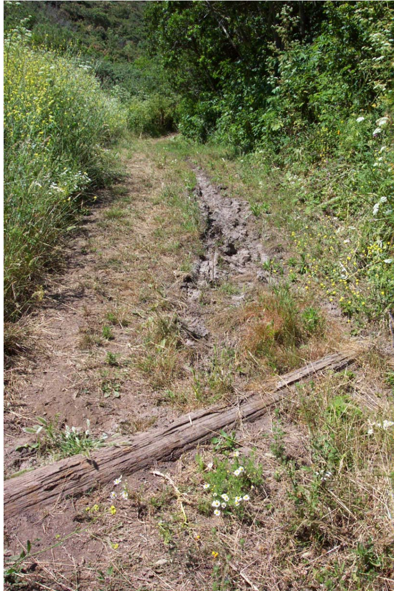
Figure 81: Incision in trail routing sediment directly into stream (Point 5 on Figure 79).
