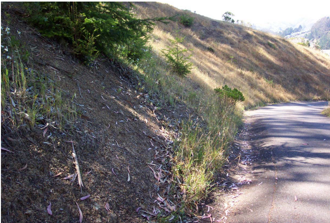
Figure 69: Surface erosion upslope from road eroding directly to drainage ditch (Point 2 on Figure 61).
