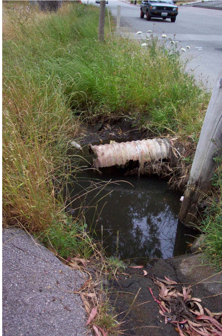
Figure 86: Channel incision from culvert draining the urbanized hillslope at Point 1 on Figure 85.
