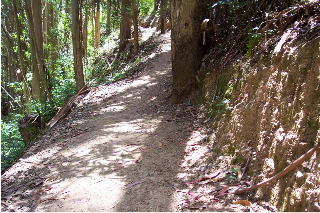
Figure 66: Surface erosion on Brooks Creek Trail with rilling in unconsolidated landslide deposits on the upper trail cut (Line 4 on Figure 61).
