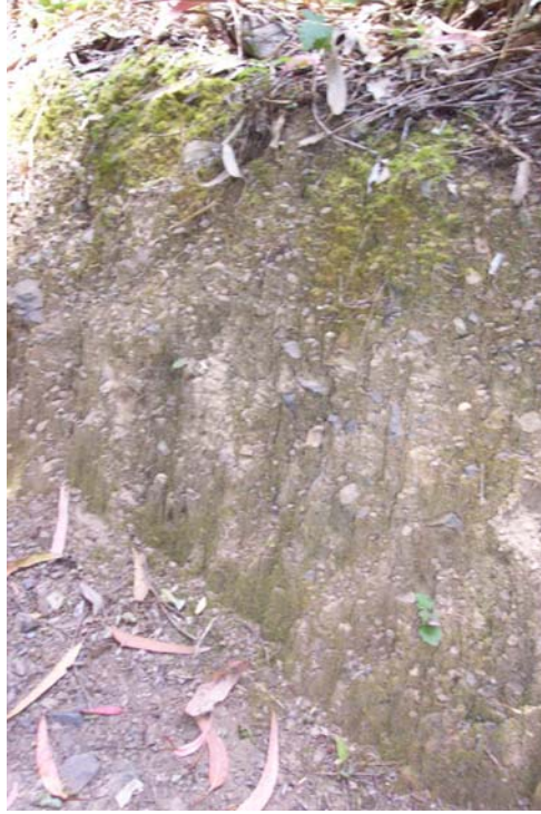
Figure 25: Rills on the nearly vertical face of an uphill trail cut in the South subwatershed.
