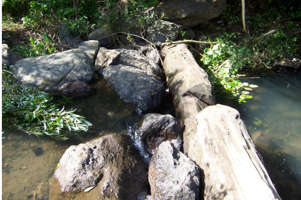
Photo 5: Undercut at Log Weir 14 at 2513 m.
