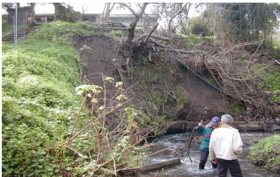
Photo 2: Bank erosion below Capistrano Bridge 2004. Photo courtesy of San Pedro Creek Watershed Coalition.
