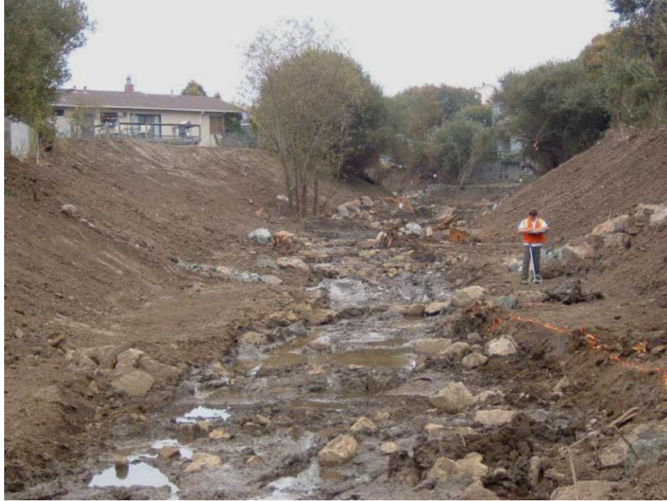
Photo 4: Intermediate weirs and bed load augmentation. Photo courtesy of Questa E.C.
