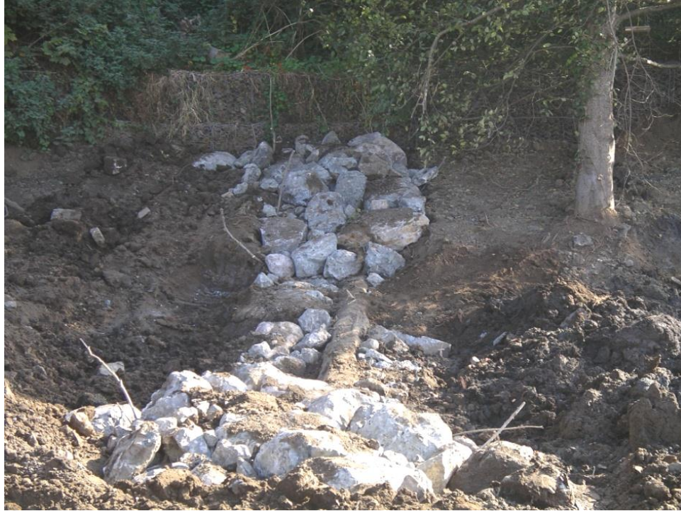
Photo 3: Completed log weir prior to backfill. Photo courtesy of Questa E.C.
