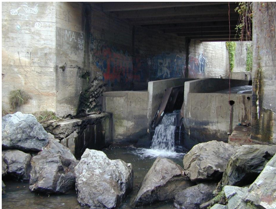
Photo 1: Capistrano Bridge Culvert and fish ladder 1999. Photo courtesy of San Pedro Creek Watershed Coalition.
