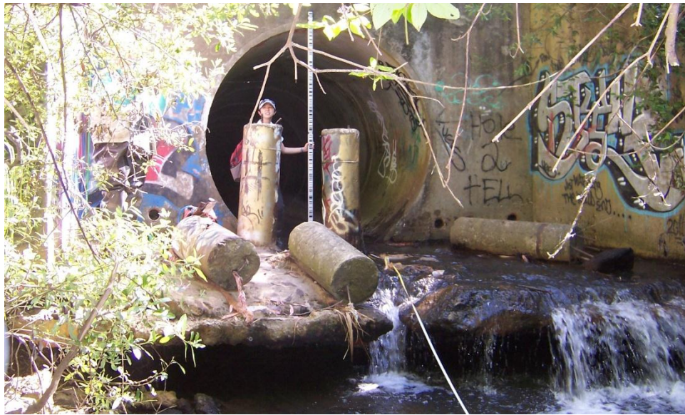
Photo 11: North Fork culvert. Eroded apron at lower center.
