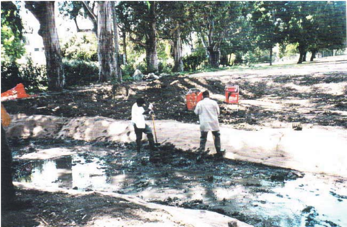
Figure 55: Brush-Layering a bank.
