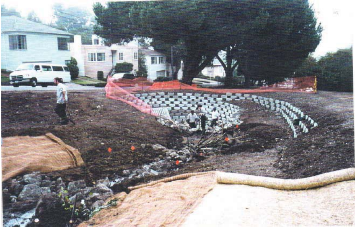
Figure 45: The 1996 daylighting of Baxter Creek in Poinsett Park used coir erosion-control fabric to achieve a more "finished" look. In the foreground of the bottom photo, the first few willow poles installed can be seen. Photos by author. 1996.
