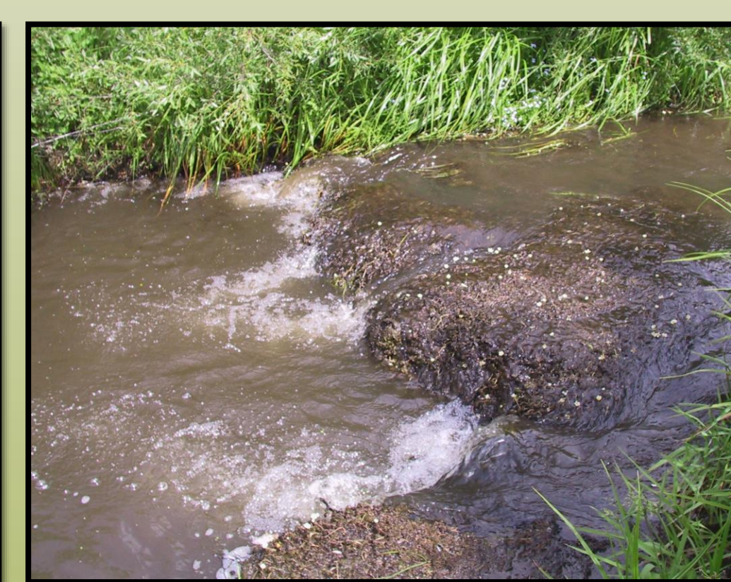
Figure 9: Longitudinal profile of a post-restoration channel near the head of Knuthson Meadow. Figure 10: Step and scour pool cut into a thickly sodded Carex -dominated wet meadow soil
