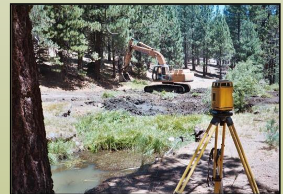
Figure 5: Example of pond and plug restoration at Two Cone Meadow (SVRCD, 2004)
