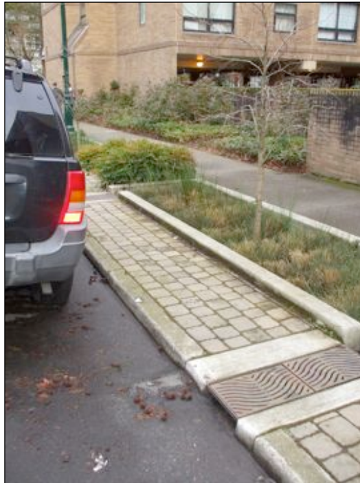
Figure 9: Flow-through planter and parking in Portland, OR. Photo by Alicia Omlid
