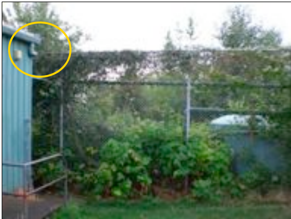
Figure 12: Disconnected downspout from building (yellow) connects to cistern (behind fence). Portland, OR. Photo: A. Omlid.
