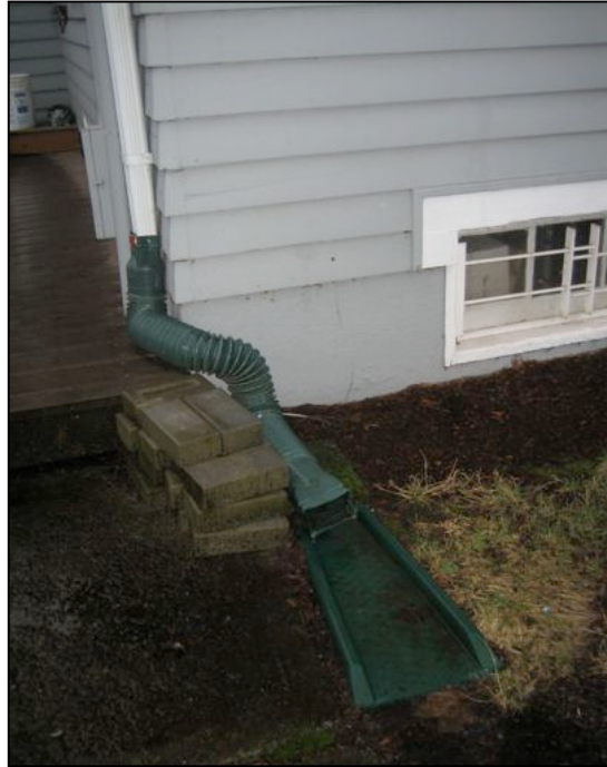
Figure 13: Disconnected downspout with dissipator (can also lead to a rain garden or, alternatively be attached to rain barrel or cistern). Photo: A. Omlid.
