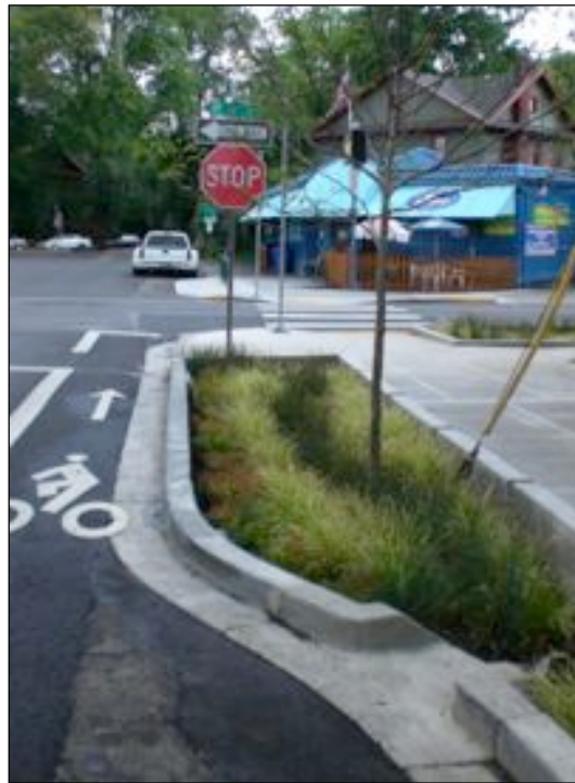
Figure 7: Curb-cut to direct stormwater into planter in Portland, OR. Photo: A.Omlid.
