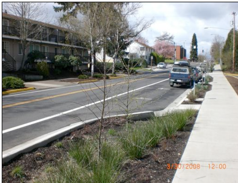
Figure 6: Flow-through planter in Eugene, OR. Photo: A. Omlid.
