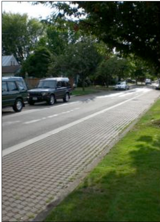
Figure 10: Permeable paving blocks in Portland, OR. Photo: A. Omlid.
