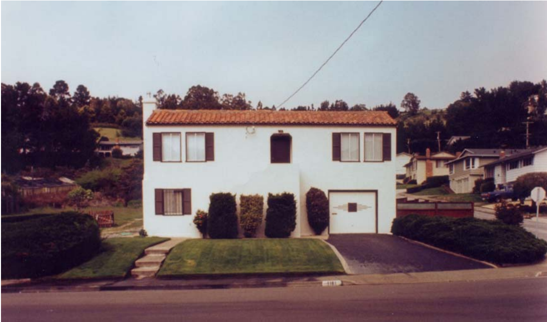
Figure 17. Malavear house on Linda Mar Boulevard (photo by author).
