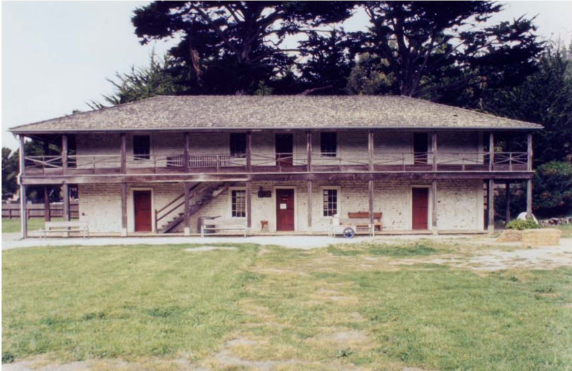
Figure 7. Sanchez's Old Adobe house as seen today at the Sanchez Adobe County Historic Site (photo by author).
